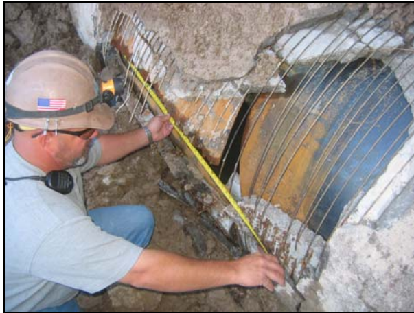
Employee assessing damage to pipe and taking measurements in preparation for the temporary repair.
