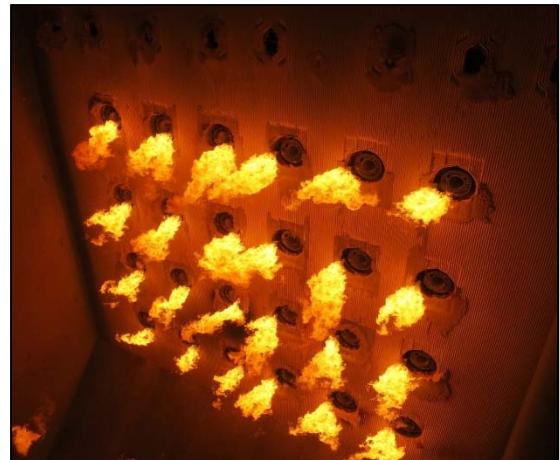
New fuel oil igniters being tested to ensure they were working properly.
