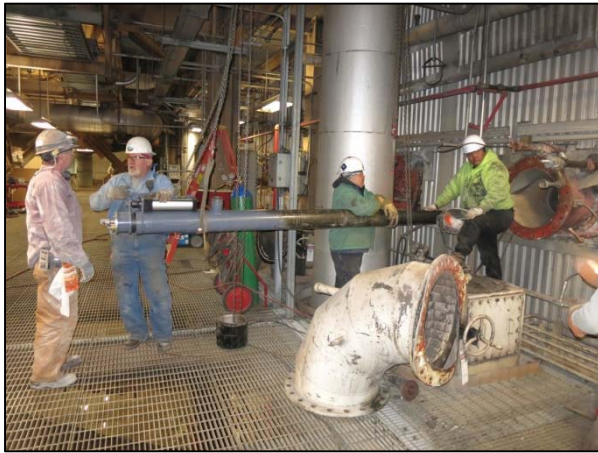
Replacing a burner oil igniter with an FPS retractable oil igniter.
