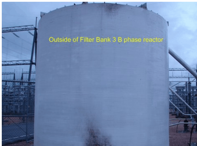
One of the filter banks damaged during a fire at the ICS AC yard.
