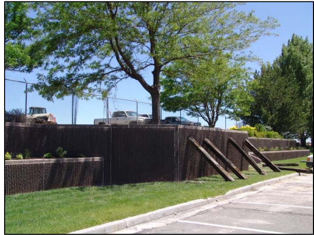
Braces were placed against the retaining wall to hold it in place until repairs could be made.
