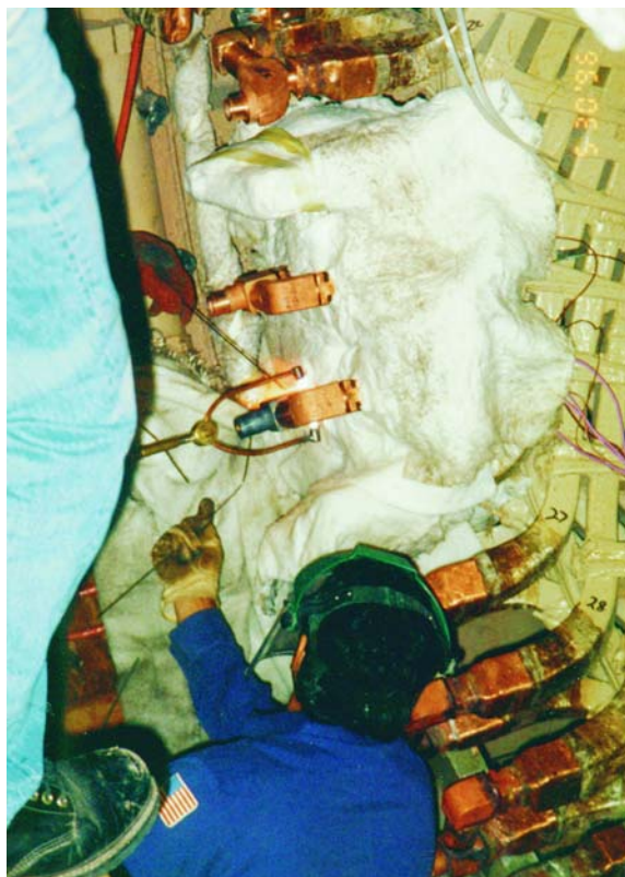
GE employees performed a generator stator bar repair.
