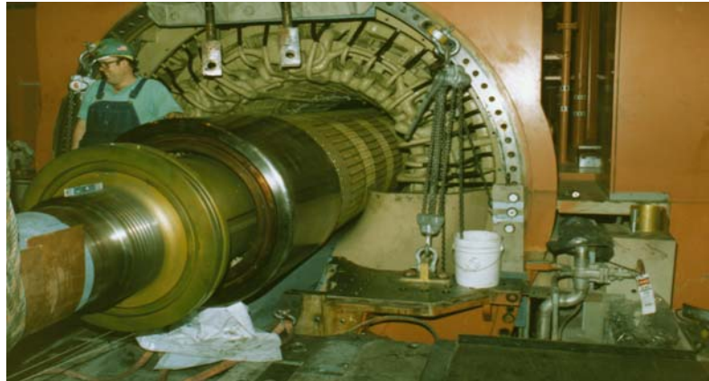
Turbine generator disassembled for inspection and repairs.
