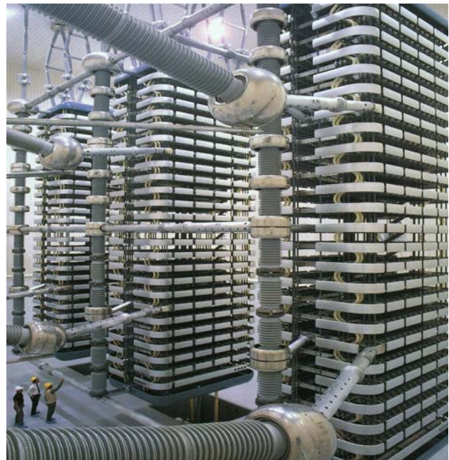
Converter Station Valve Hall.
