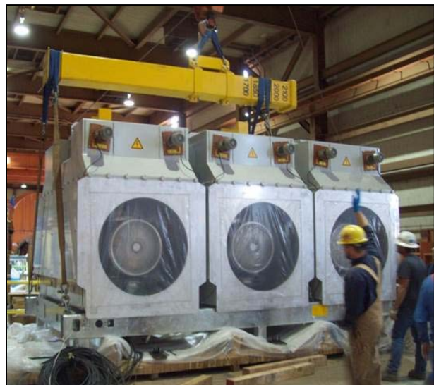
New breaker getting ready to be installed.
