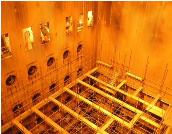
Scaffolding being erected in the boiler.
