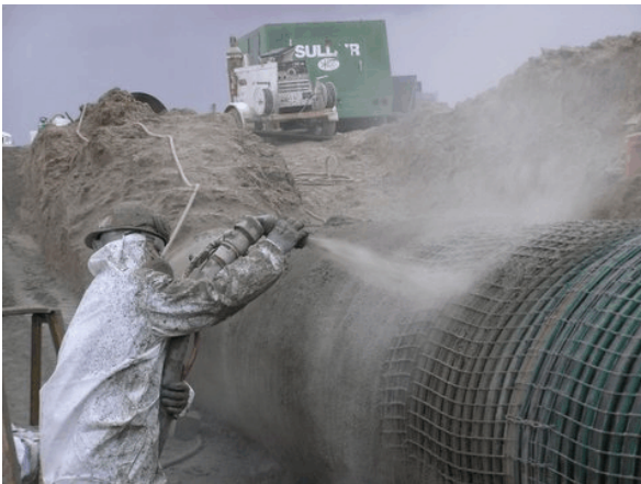
Employee spraying Guniting (cement-like material) over pipe wrapped in mesh fencing.
