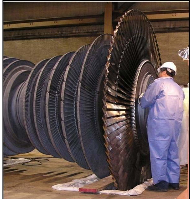
Unit 2 LP Turbine - last stage bucket installation of new buckets.
