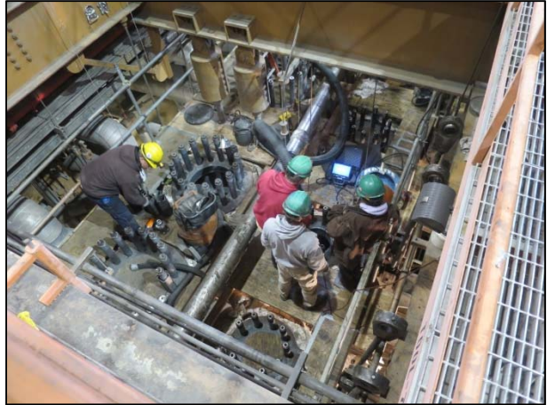
IPSC employees swapping out turbine stop and control valves.
