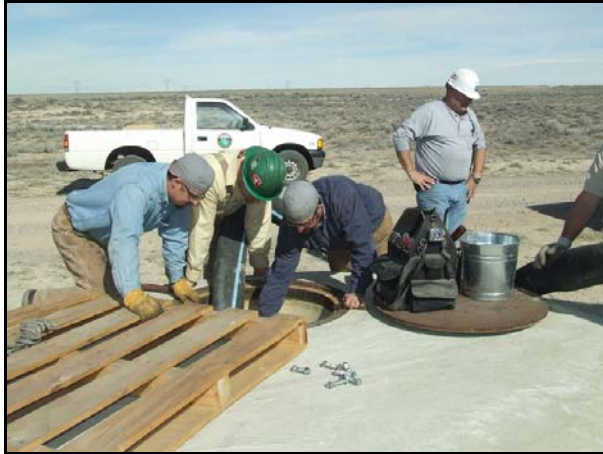
IPSC employees and contractors lowering the RFEC/TC into the DMAD pipeline.
