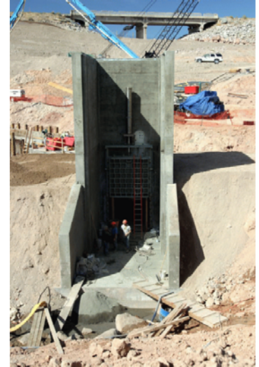
Tower outlet guard gate.
