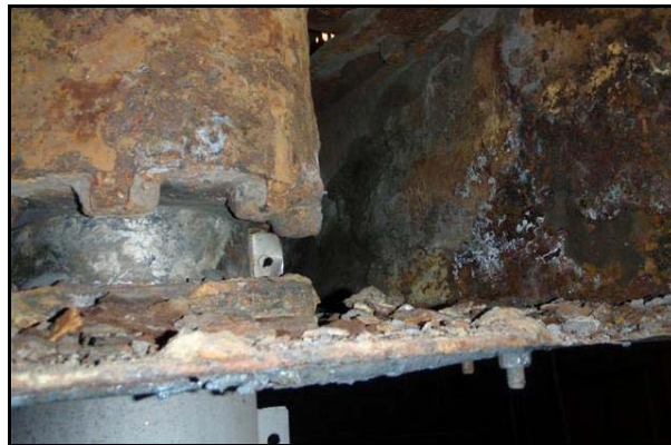
Extensive corrosion underneath the reaction tank mixer gearbox. This picture shows a support beam on the right and the mixer shaft coupling on the left.
