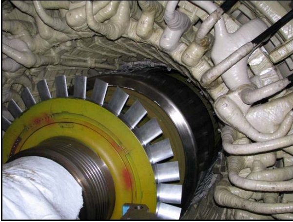
Preparing to remove Unit 2 generator rotor.
