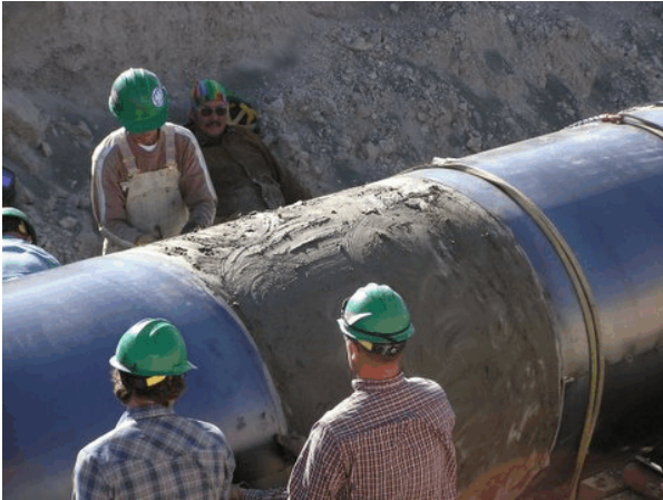
Employees preparing the pipe to have the sheet metal wrapped around it.
