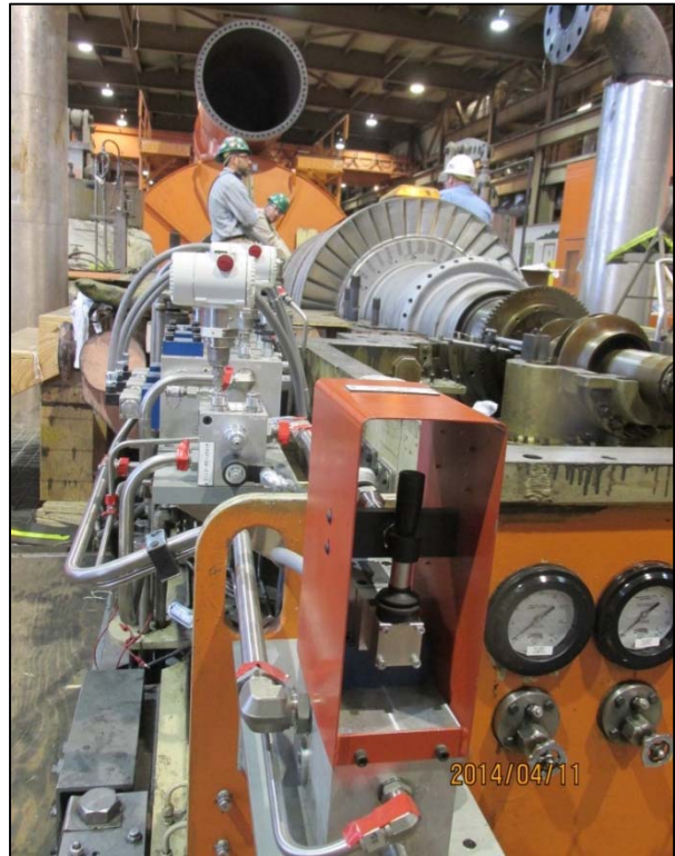
Employees working on the Turbine Over-Speed Trip Replacement.
