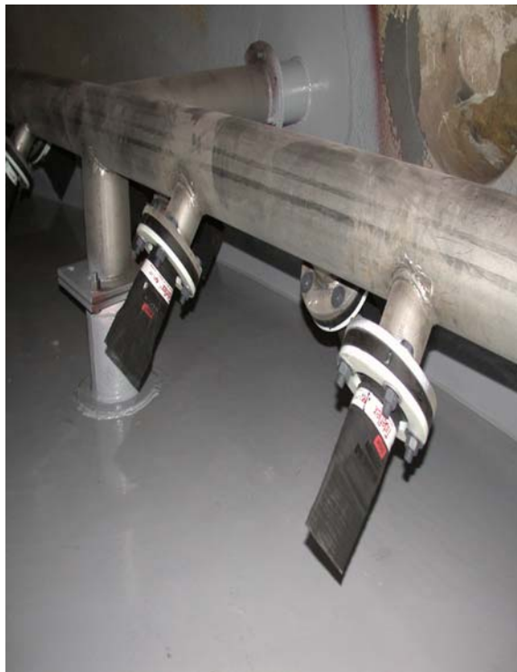
Sparger nozzles added to four of the reaction tanks in Unit 1. This will provide air for forced oxidation.
