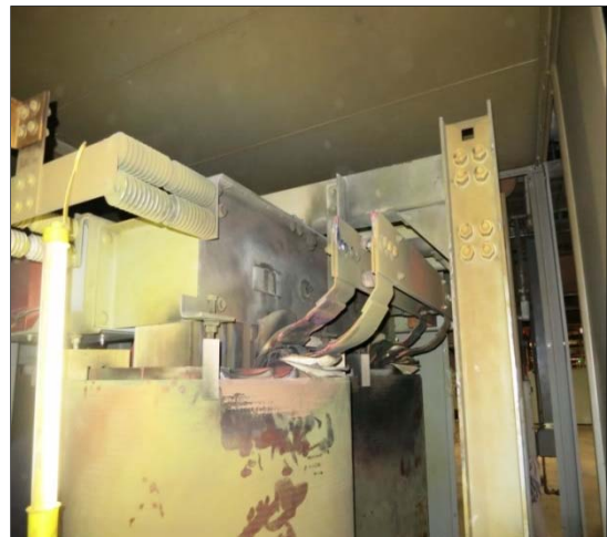
Failed C Phase of the Generator Excitation Power Potential Transformer.
