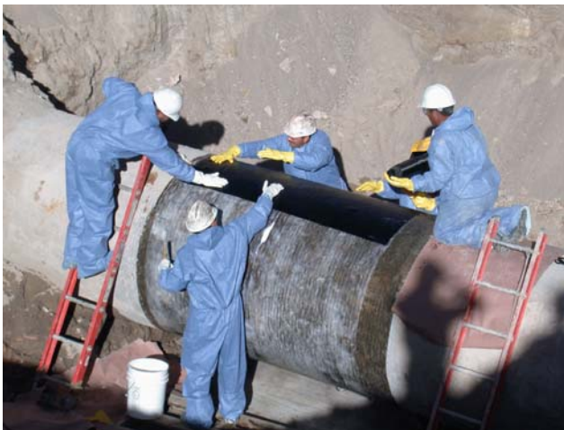
Contractors fixing a leak in large pipe that comes from DMAD Reservoir.
