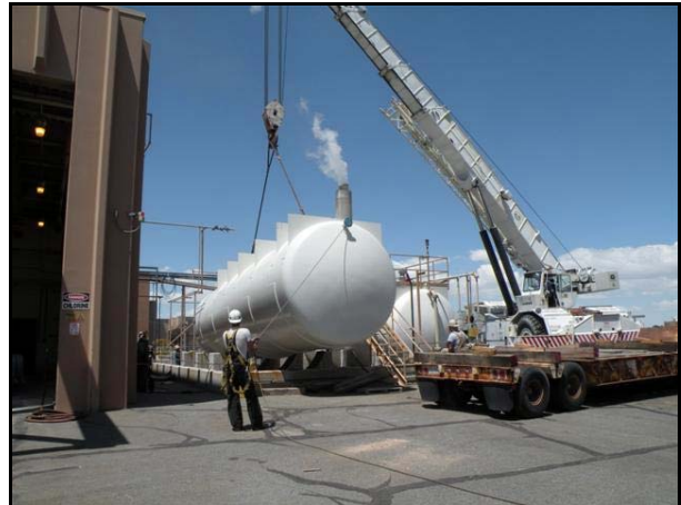
The new acid tank being installed.
