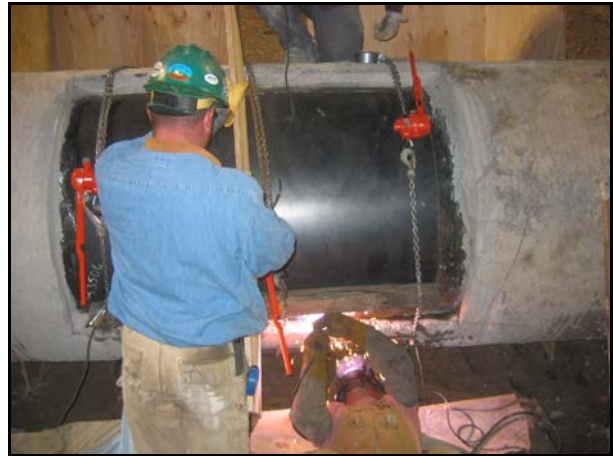
Employees welding steel pipe replacement in broken section of pipe.
