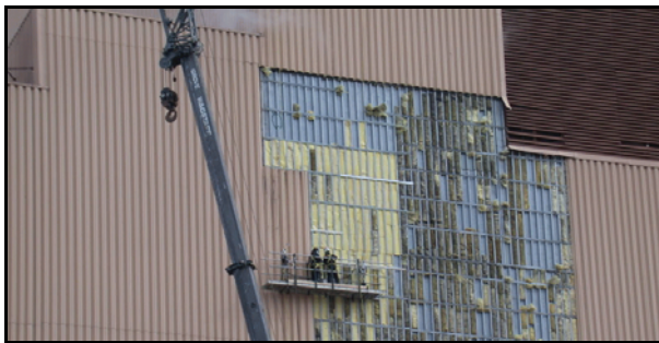
Installing siding on the Unit 2 Boiler building.
