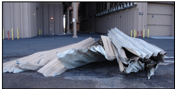
Siding torn off of the Unit 2 Boiler building by strong winds.
