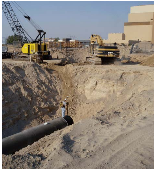
Surface water supply line replacement.
