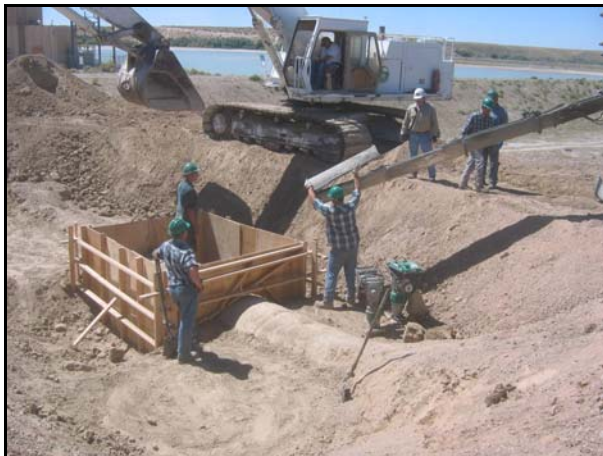
Employees preparing to pour cement for the temporary pipe repair.
