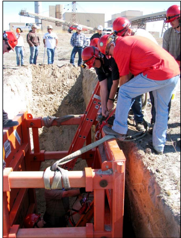
Rescuers beginning to lift patient out of trench box.
