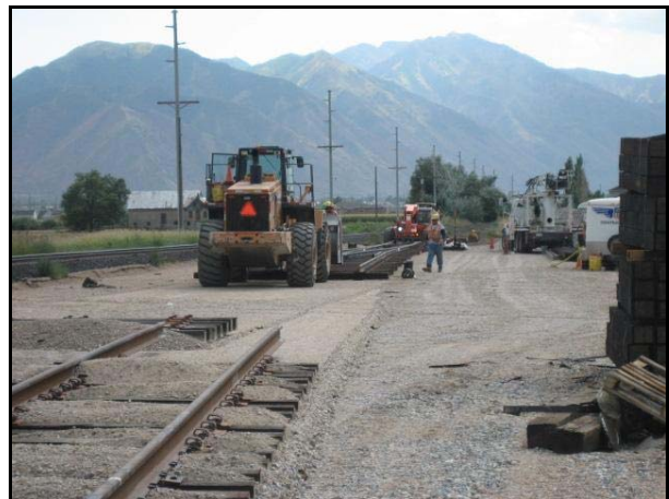
Placing ties and rails for the new track #4.
