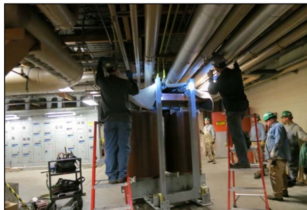
Generator Excitation Power Potential Transformer being moved under overhead piping.
