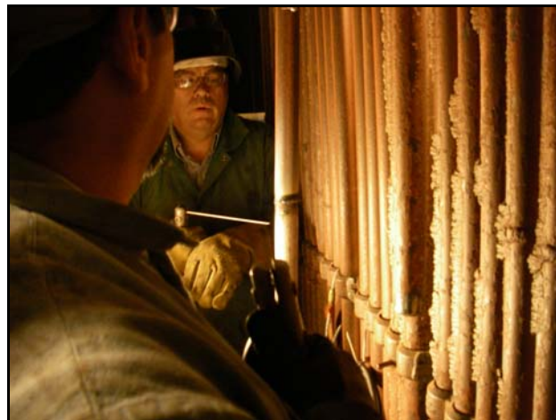
Employees repaired boiler tube leaks on Unit 2.
