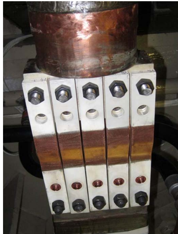
The new generator terminal connection.
