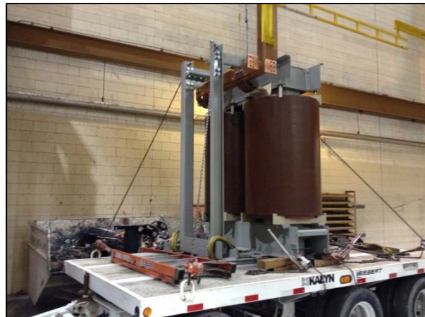
New Generator Excitation Power Potential Transformer.
