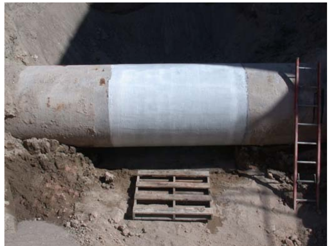
Completed wrap on pipe to repair leak.
