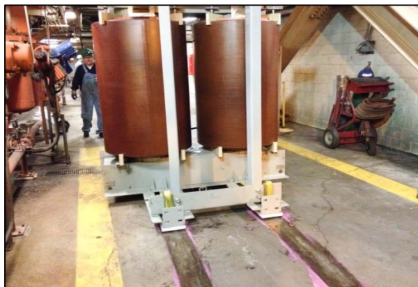
Generator Excitation Power Potential Transformer being moved on skids covered with dish soap.
