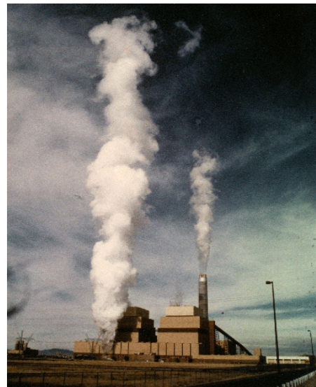
Steam blow of the boiler.
