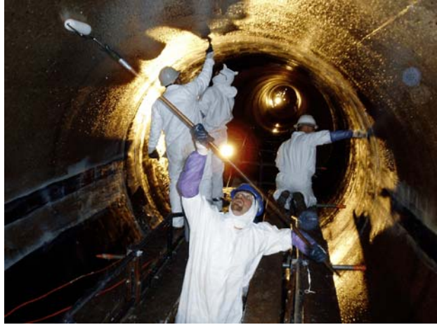
Reinforcing circulating water lines with carbon fiber.
