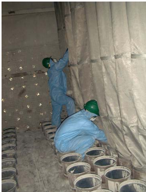
IPSC employees replacing filter bags in the baghouse.
