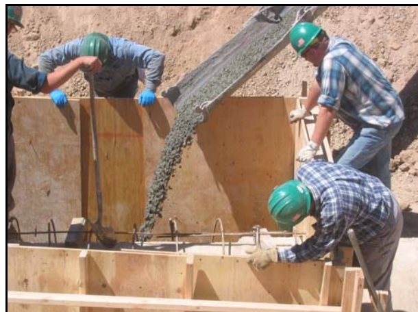
Cement being poured into forms for the temporary pipe repair.
