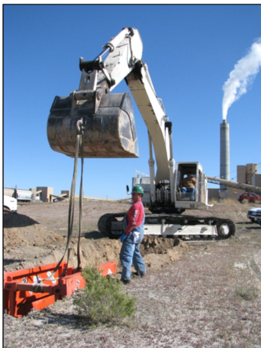
Backhoe lowering trench box into the trench that was dug.
