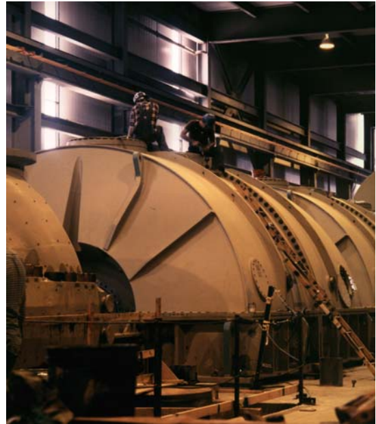
Construction of the turbine generator.
