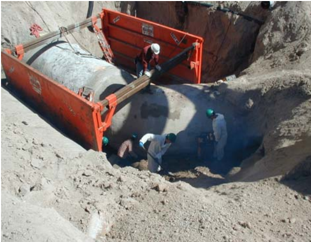
Employees working on the Cooling Water Pipeline Repair
