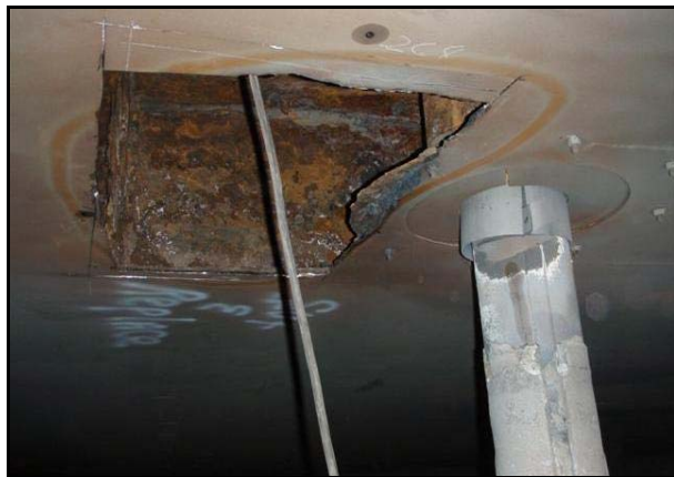
Hole cut in reaction tank ceiling to remove corroded and thin spots.
