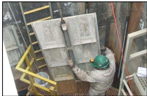
Installing one of the Riser Gates in the Cooling Tower.
