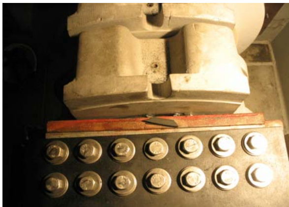
Ruptured gasket at the top of the X1 bushing.
