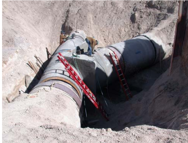
Underground pipe being worked on to repair leak.
