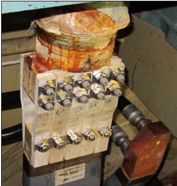
Original generator terminal connection.
