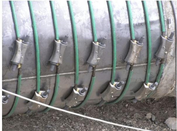
Tension bands wrapped around pipe.
