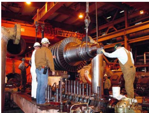
Employees installing high-pressure turbine.
