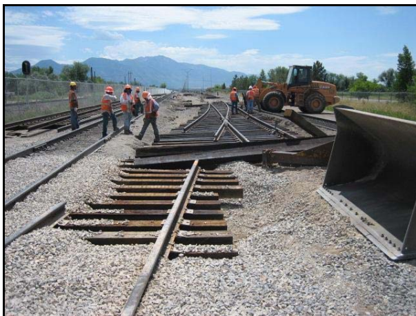
The extension and addition of railroad tracks in the Springville yard required several new switches be installed.
