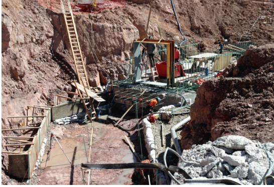
Construction of new outlet pipe.
